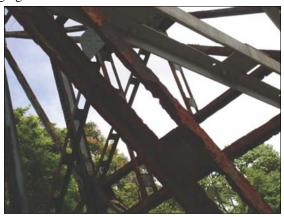
Weather permitting, spraying will begin at the end of February and continue in two phases. The process will consist of an initial inhibitor application, including time allowed for saturation to counter the buildup of corrosion scale, followed by a second application within hours of the first. The specification is to spray the bridge annually until the budget allows for the complete replacement of components, after which a conventional coating system will be put into place.
